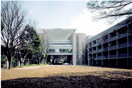
美術学部総合工房棟 Factory Complex (A), Faculty of Fine Arts
