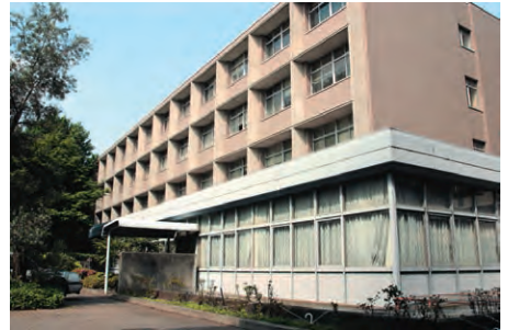
音楽学部5号館 Building V, Faculty of Music
