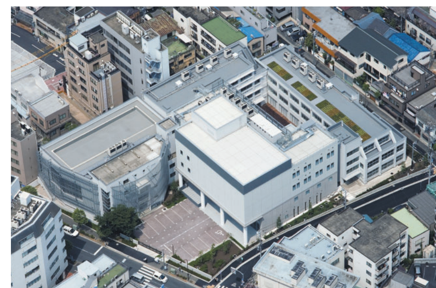
① A棟 Building A
